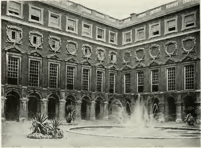
189. Fountain Court, Hampton Court Palace.
